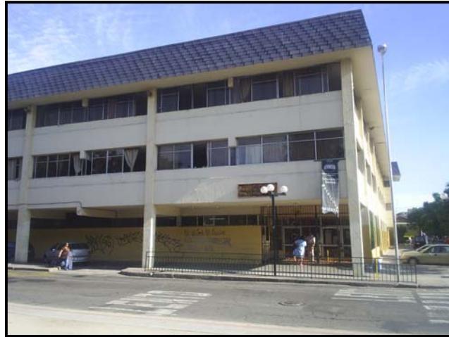
Fachada principal del colegio (Agustinas/García Reyes)
