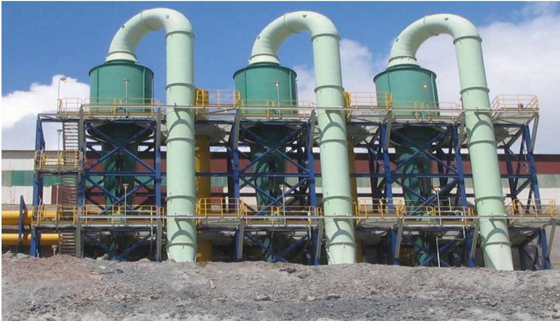
Fig. 33: Sistema Colector de polvo Aeromix Wet Scrubbers.
